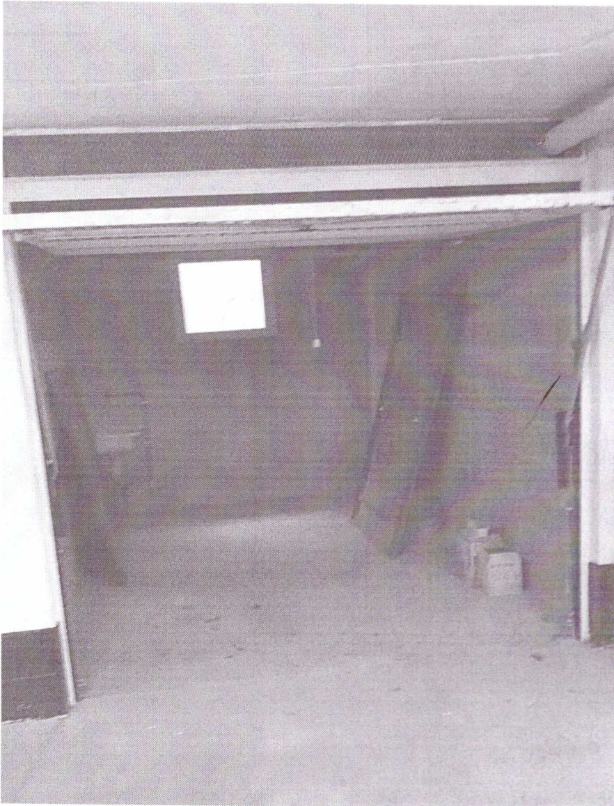
Foto 30 – Garage, Fg 8, part 318, sub 8.
