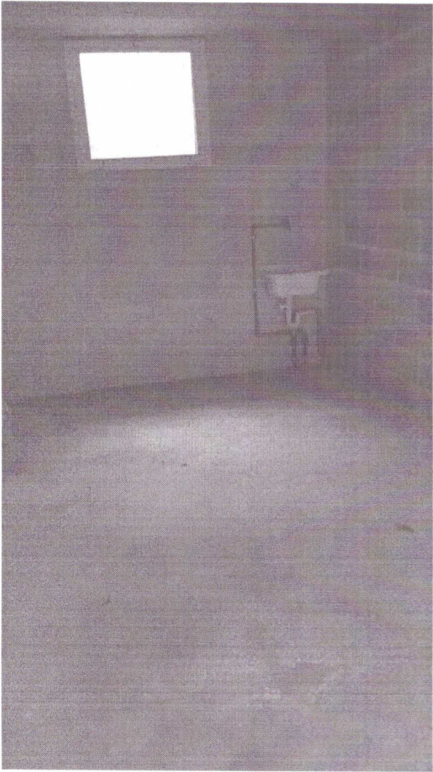
Foto 20 – Garage, Fg 8, part 318, sub 7
